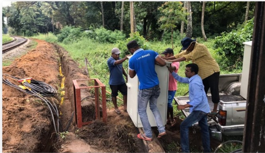
Placing a Cabinet at Dambegoda
